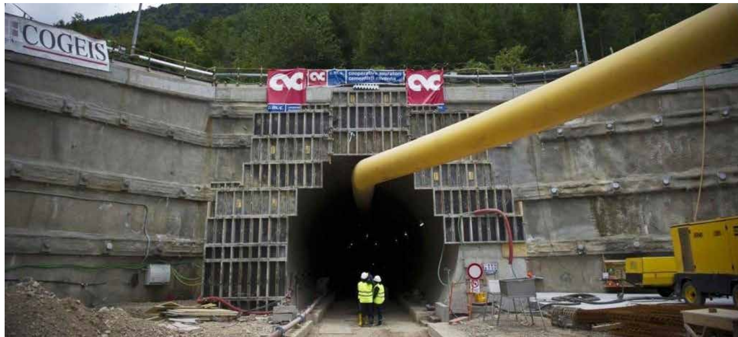
Drilling operations and the entrance of the construction site of Chiomonte geognostic tunnel
